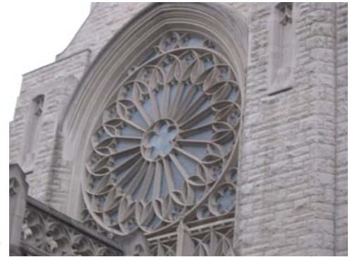
The facade window at Sacred Heart Parish in Shadyside will be among the architectural features of the tour.
